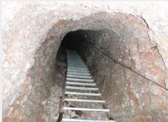
Ulaz u tunel
